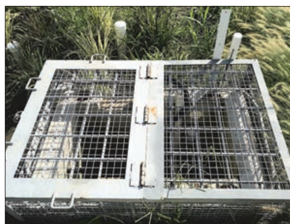
A flow monitoring station at the rain garden. Previously PennDot would have simply installed concrete detention basins, which can overflow.
