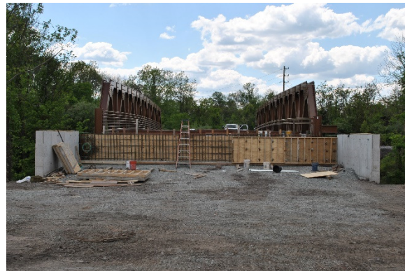
Figure 1. Existing and Reconstructed Paradise Street Vehicular Access – New Deck Raised 6 Feet Above Existing
