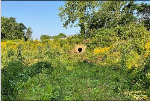
Figure 2. 54" stormwater outfall from high school parking lot discharging into preformed scour hole with level spreader to floodplain design.
