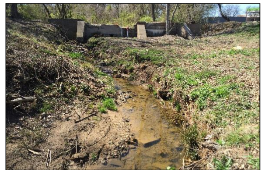
Figure 1. Existing concrete dam structure impairing aquatic organism passage and river continuity.
