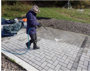
Power Washing Before Applying a Shop Vac
