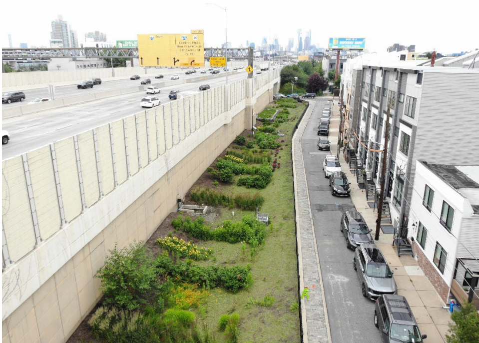
Figure 1. Experimental bioinfiltration basin that receives saline stormwater runoff from I-95 in Philadelphia.
